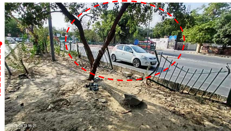
Median opening due to damaged guardrail, people tends to cross the road from median which making pedestrians vulnerable
