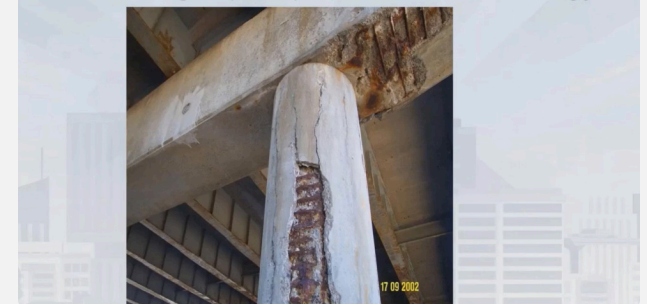
Corrosion damage of pier caps and columns due to leaking joints
