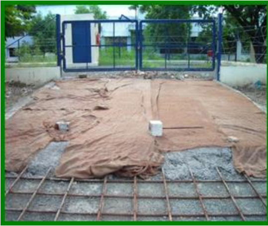
(a) During construction (2010) Fig. 7 GPC road at CSIR-SERC Campus
