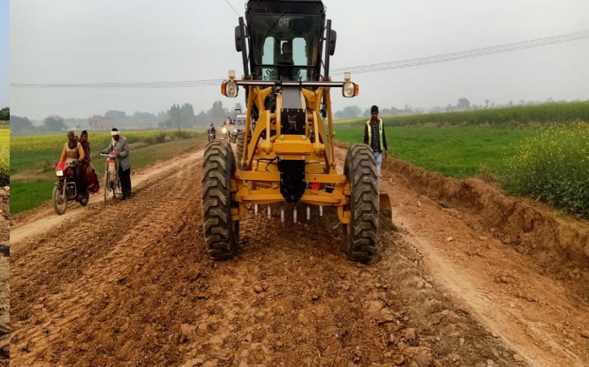
8. Grading and Mixing with Grader
