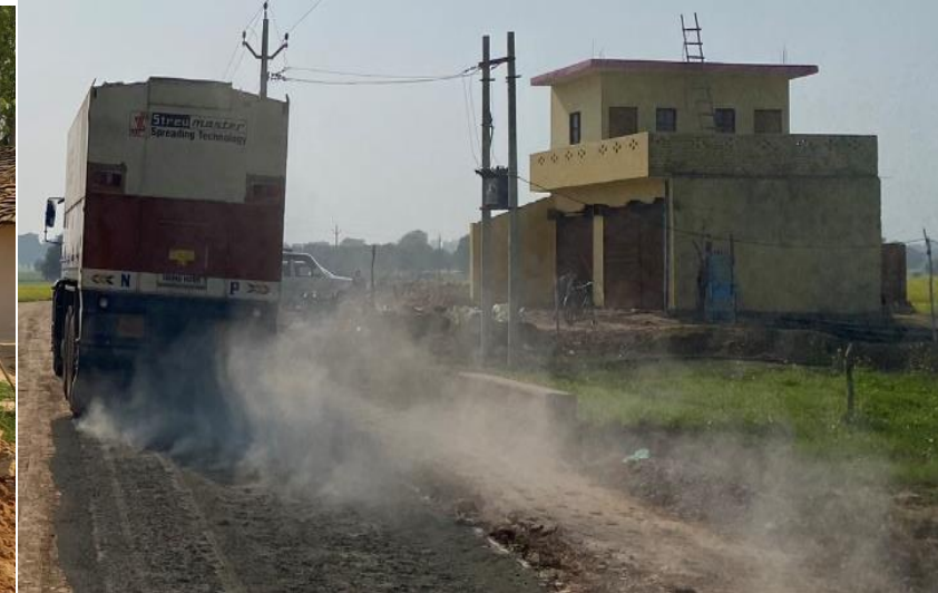
5. Cement Spreading with Spreader
