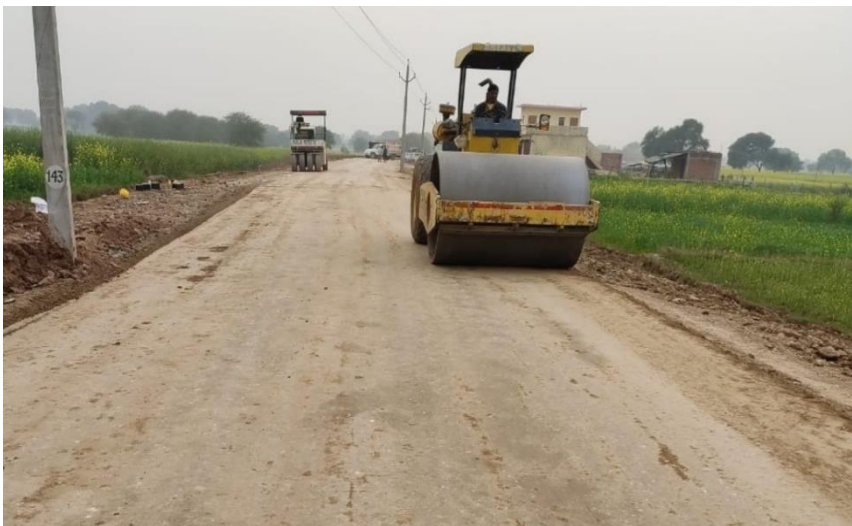
9. Compaction with Vibro Roller
