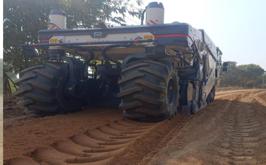
2. Scarification with Recycler
