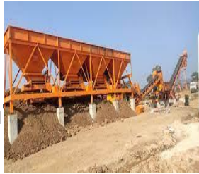
Preparation of Mix
