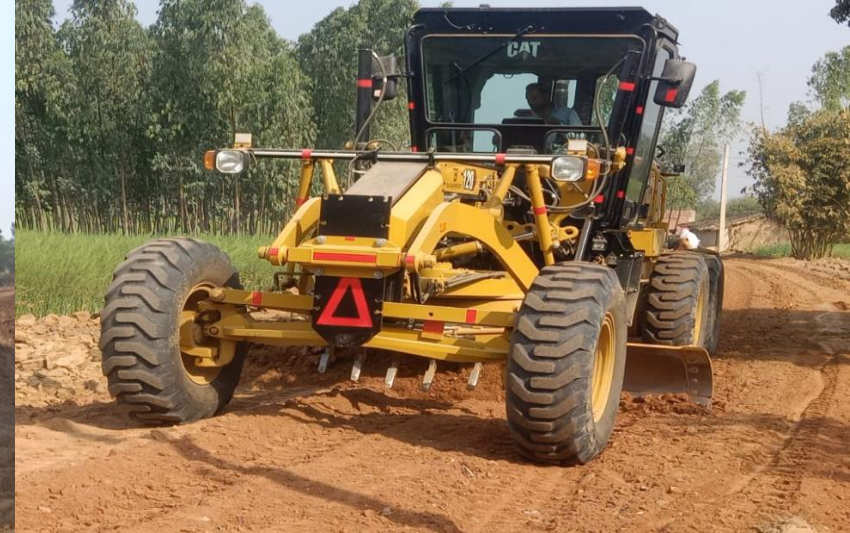
3. Grading and Mixing with Grader
