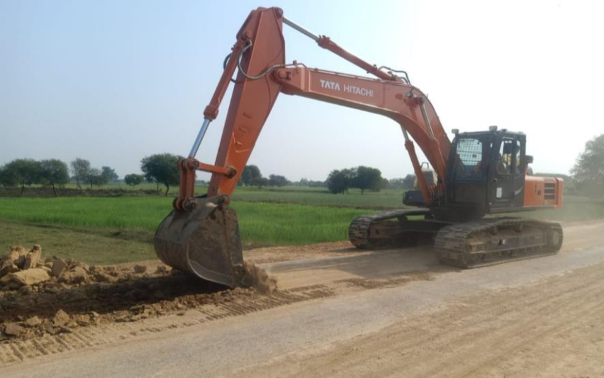
1. Shoulder Excavation & Material Removal
