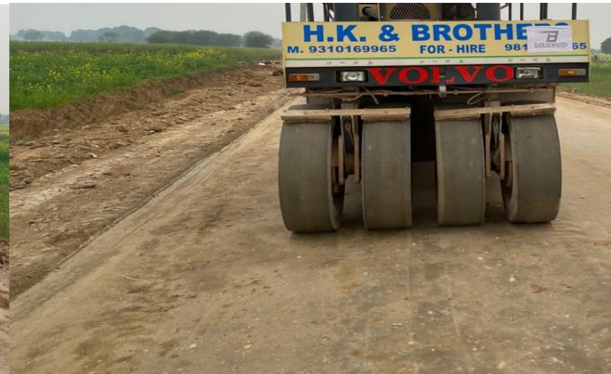
10. Compaction with PTR
