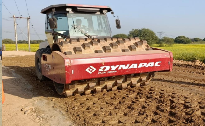
7. Compaction with Pad Foot Roller
