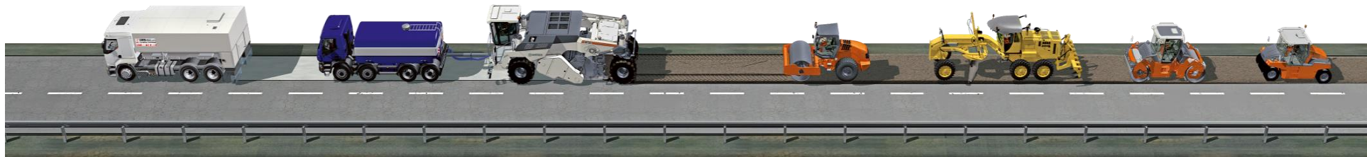
Cement/ Additive Spreading
