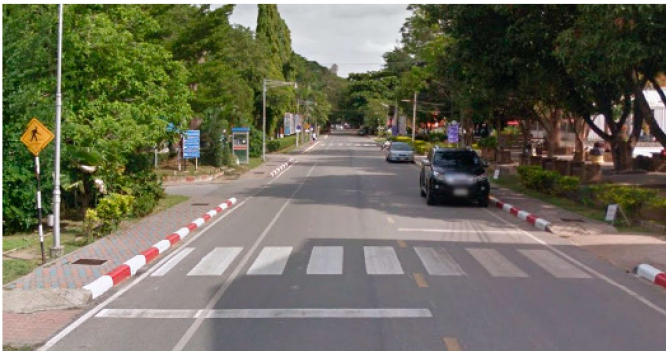
Safety issue: Miscommunication
