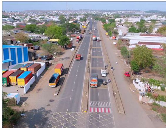
Drone Shot: Post application of safety measures at Wadhamna Intersection
