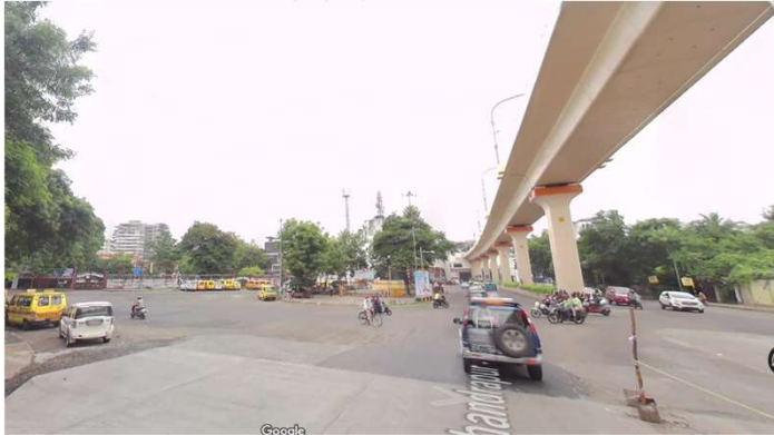
Improper traffic and pedestrian movements
