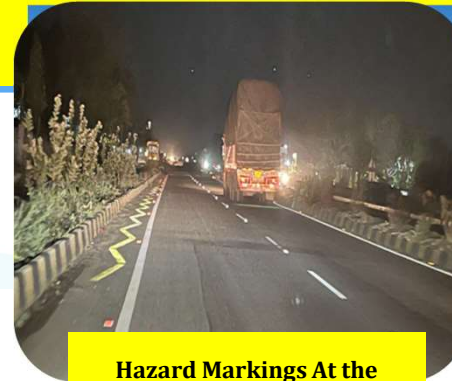
Hazard Markings At the Intersection Approach
