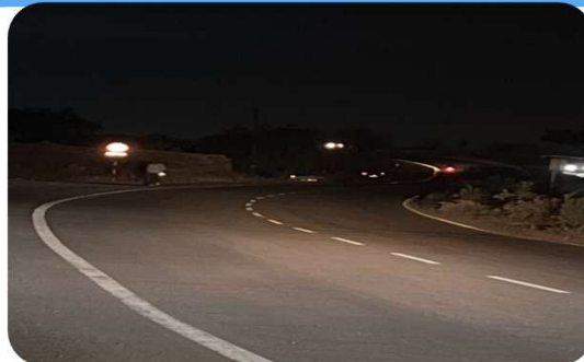
📍 Horizontal Curved section, 900 m away from the Wadhamna Intersection @ NH 53 @ Surabardi.
