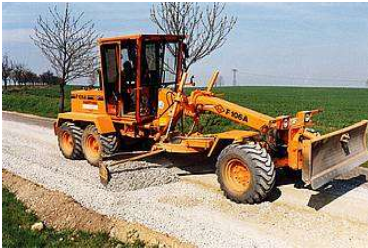
Building of self-hardening road pavings
