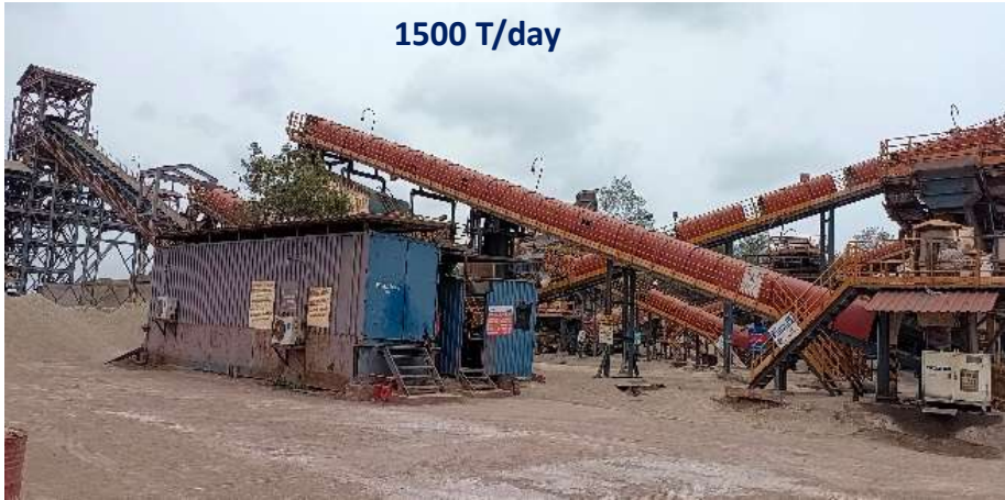
Iron slag sand manufacturing unit
