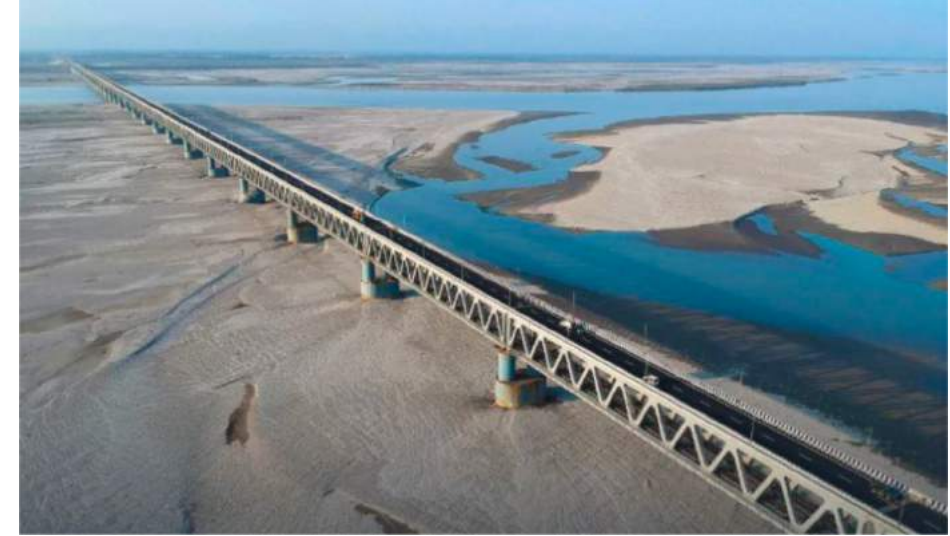
Bogibeel Bridge, Assam- 125m
