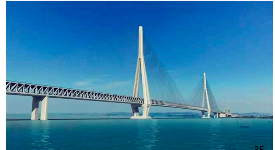
Changtai cross-river bridge, 1176m
