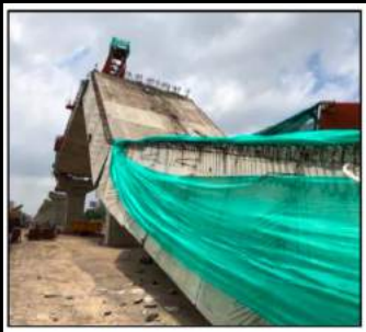
Elevated Viaduct, Haryana - 1 22.08.20
