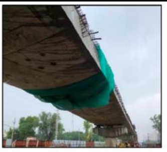
Elevated Viaduct, Haryana - 2 15.07.20
