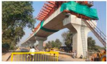
Elevated Viaduct, Varanasi November 2018
