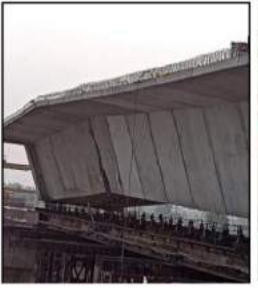
River Bridge, Haryana - 1 19.06.19
