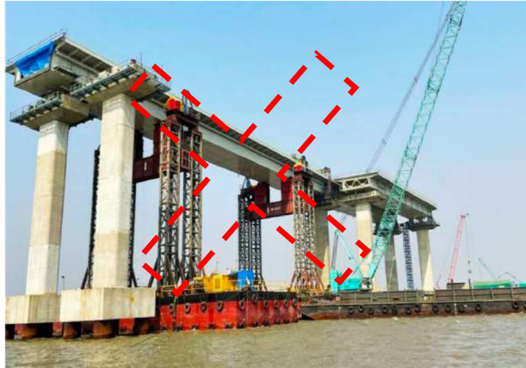
Mumbai trans-harbour link, Mumbai
