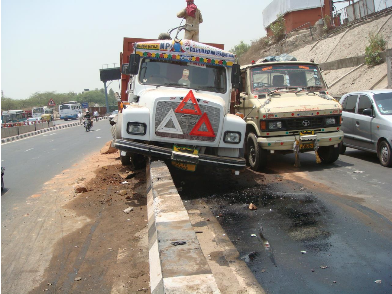
Fault of Road Agency
