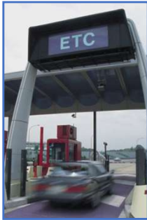
Electronic Toll Collection System
