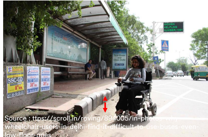
No ramp to access the bus stop / footpath
