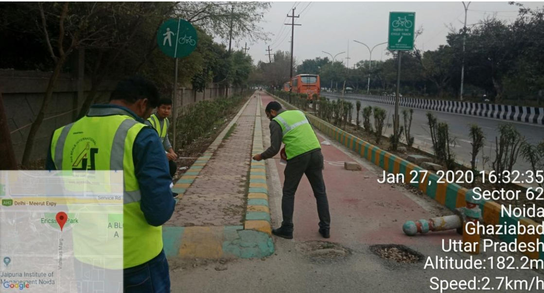
Lack of maintenance of bollards
