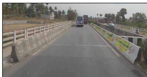
*During Audit, it has been observed that OHM sign board was missing at both end of MNB.*
