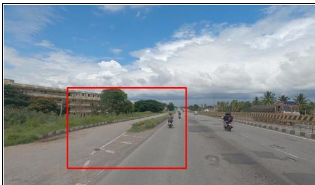
During Audit it is observed OHM sign board is missing
