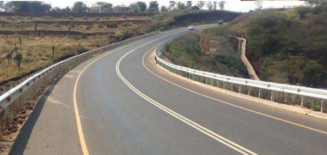
Arusha Bypass 2-Lane with Paved Shoulders (Greenfield)
