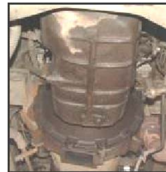
Gear box oil leakage
