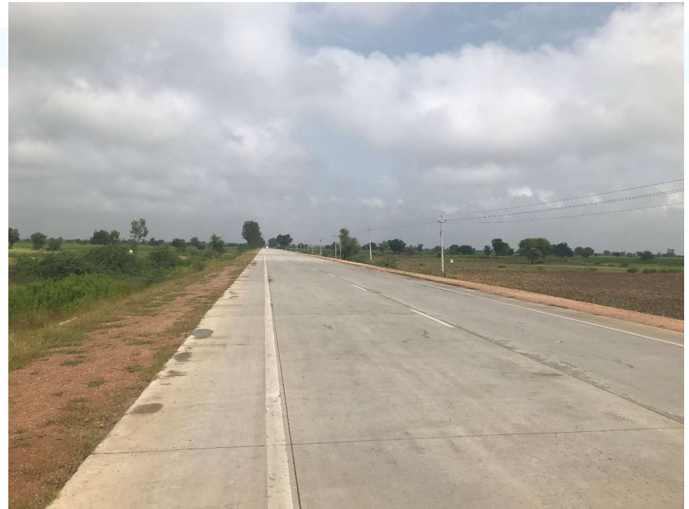
Conventional Concrete Pavement panel 3.5 m X 4.5 m with complete new crust
