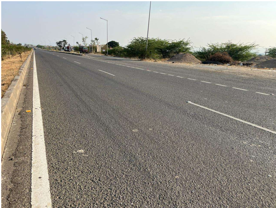
Typical pavement condition where White Topping can be implemented
