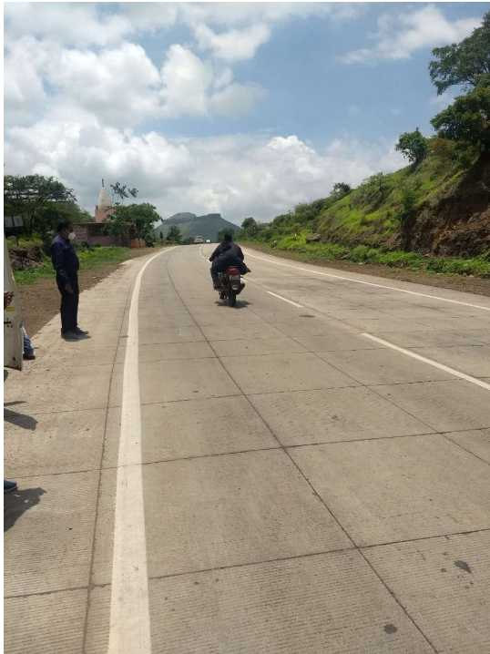
White Topping overlay 1.0 m X 1.0 m panels above existing bituminous surface
