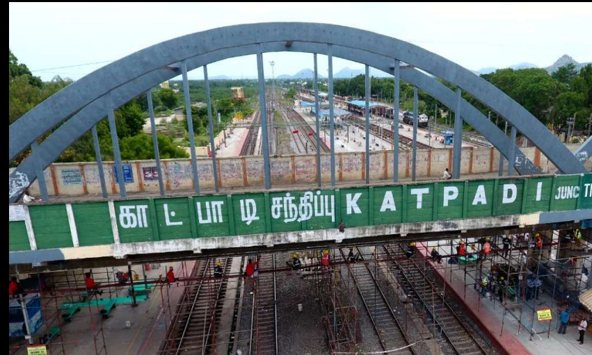
Application of Anti Carbonation aliphatic acrylic coating
