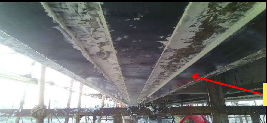
Carbon laminate after Prestressed
