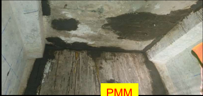
Sealing of crack with resin
