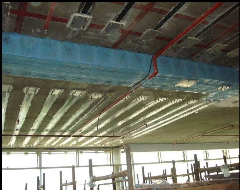
Anchor plate system
