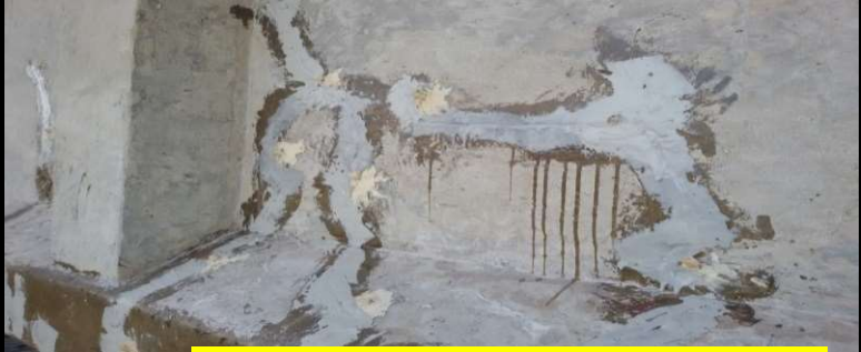
Sealing of crack with resin
