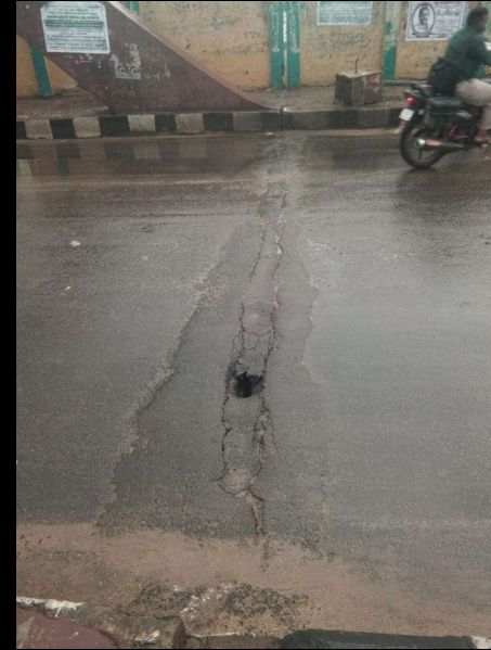
Condition of expansion joint.
