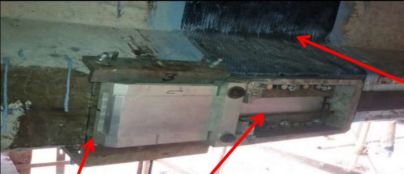
Strengthening at concrete location before prestressed begin
