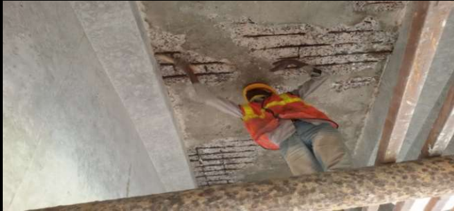
Cleaning Reinforcement
