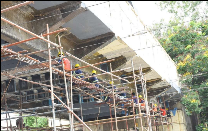
Application of Pre-stressed laminates
