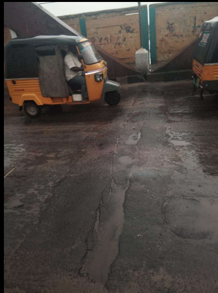
Condition of expansion joint.
