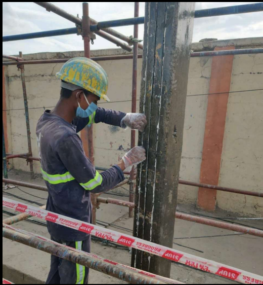
Providing Groove laminate in Hangers
