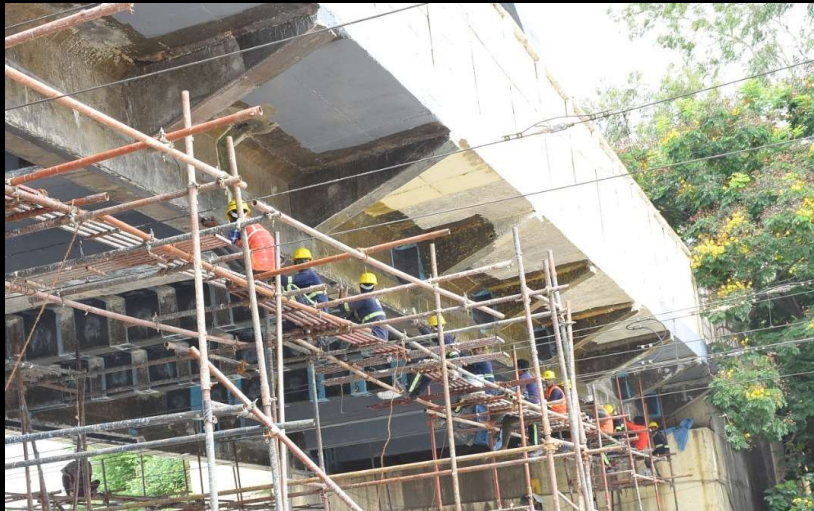
Application of Pre-stressed laminates
