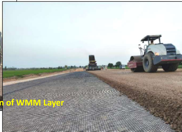
Placement of Biaxial Geogrid Layer over Prepared GSB
