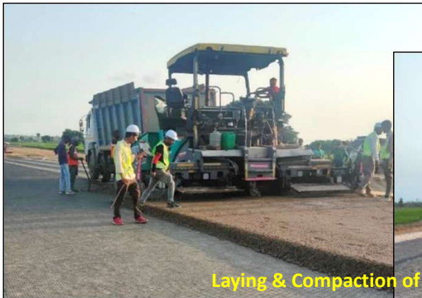
Preparation of GSB for Placement of Geogrid
