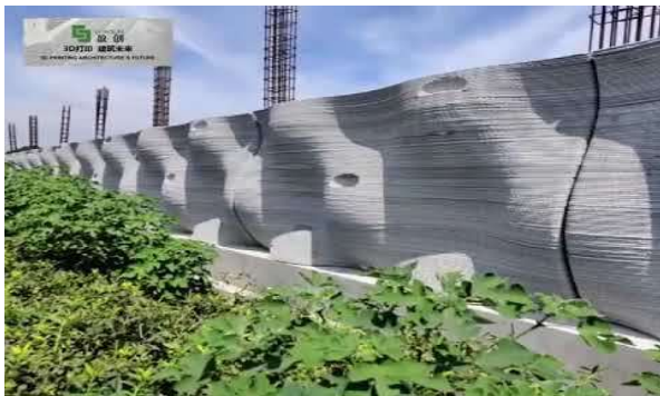
3D printed sound barriers, China
