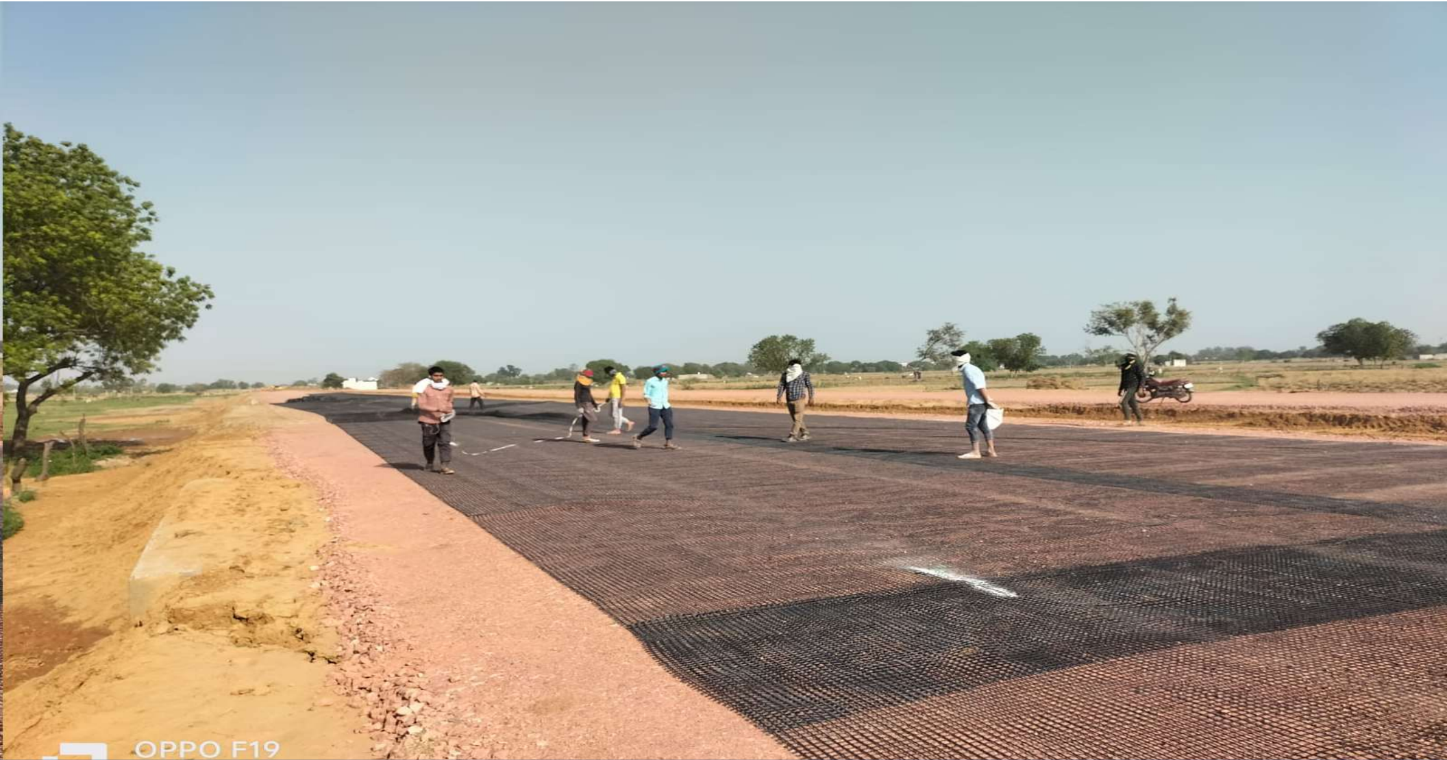
PAVEMENT STABILIZATION USING BIAXIAL GEOGRID AT LUCKNOW KANPUR EXPRESSWAY, UP
