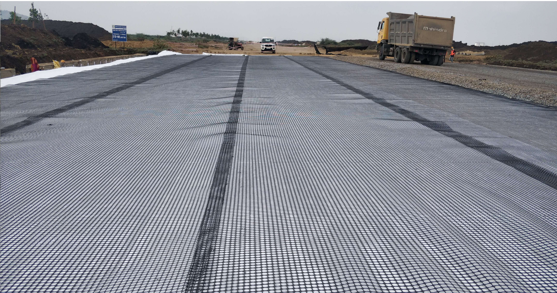
PAVEMENT STABILIZATION USING BIAXIAL GEOGRID AT AMARAVATHI, AP
