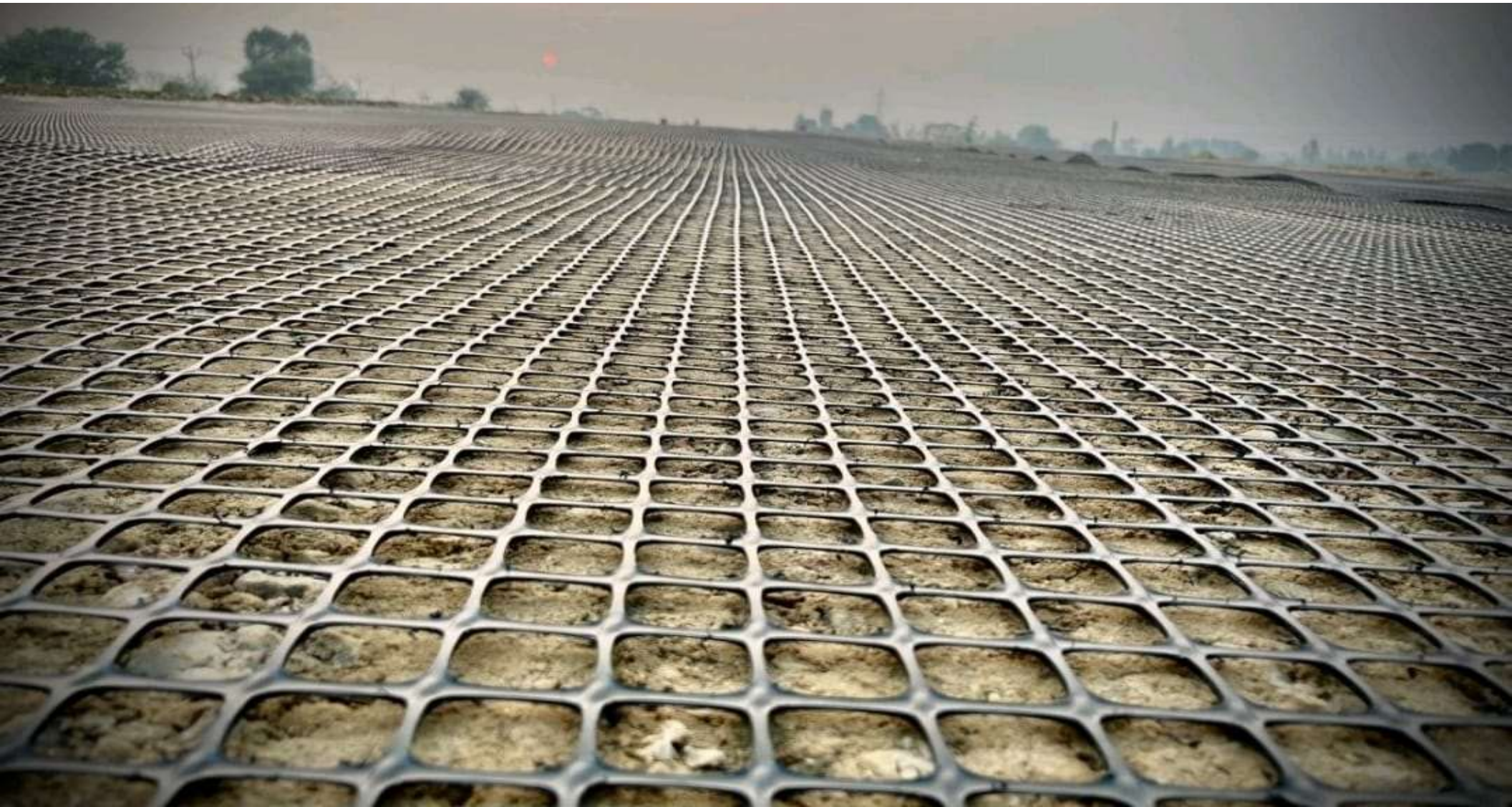
PAVEMENT STABILIZATION USING BIAXIAL GEOGRID AT RUPNAGAR, PUNJAB
