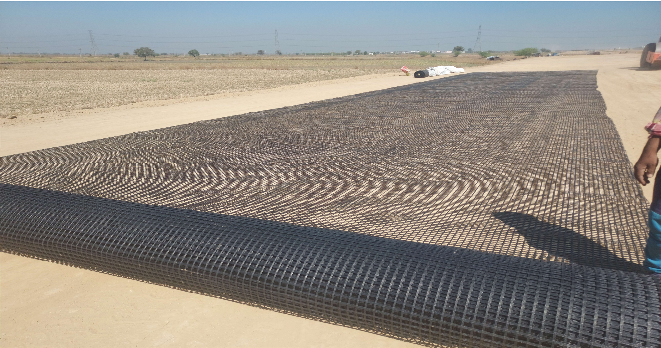
PAVEMENT STABILIZATION USING BIAXIAL GEOGRID AT DHOLERA EXPRESSWAY, GUJARAT
