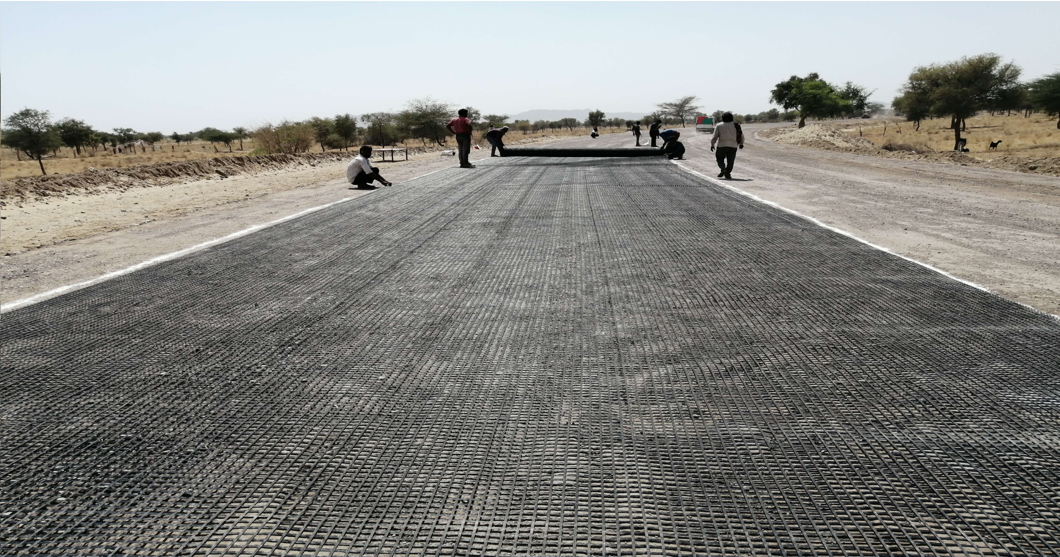
PAVEMENT STABILIZATION USING BIAXIAL GEOGRID AT BARMER BYPASS, RAJASTHAN
