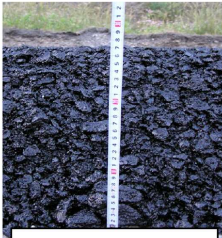
280 mm lift after Laydown
