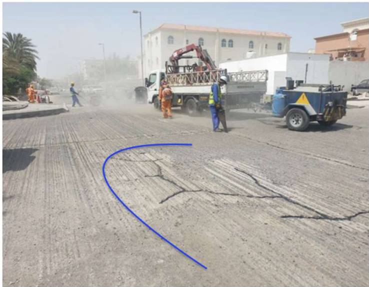
Cracks after removing asphalt layer by milling-Actually it was created during co
