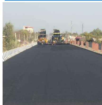
Laying of HiMA
