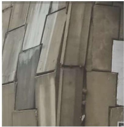
Adoption of improper construction practice, leading to poor compaction at abutment and long-term volumetric changes
