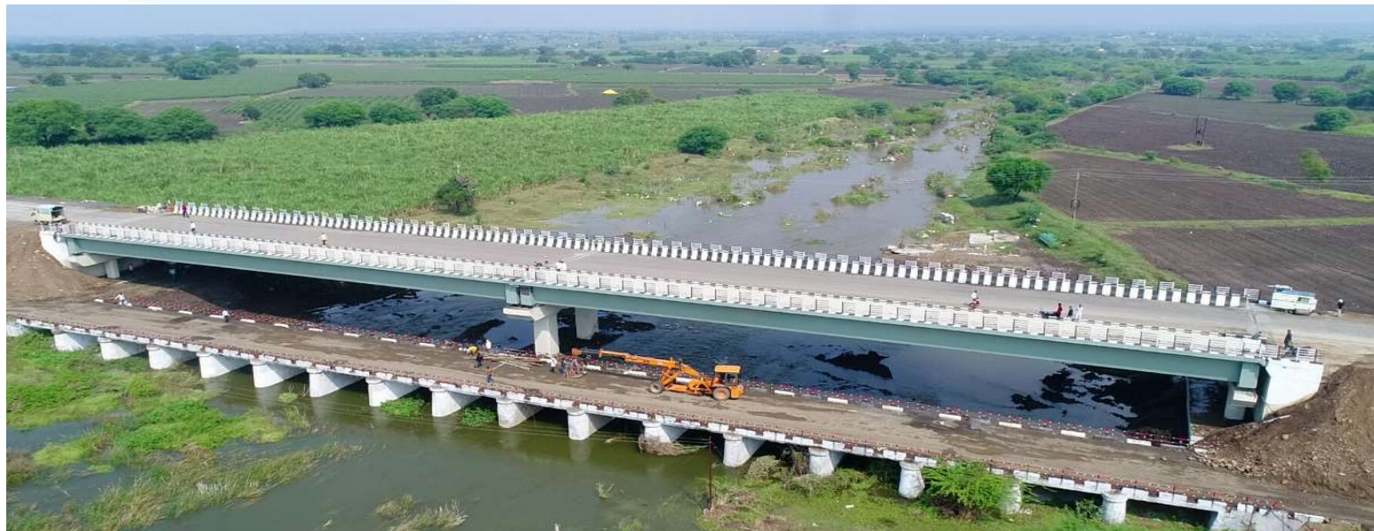
Completed Photo of Bridge
