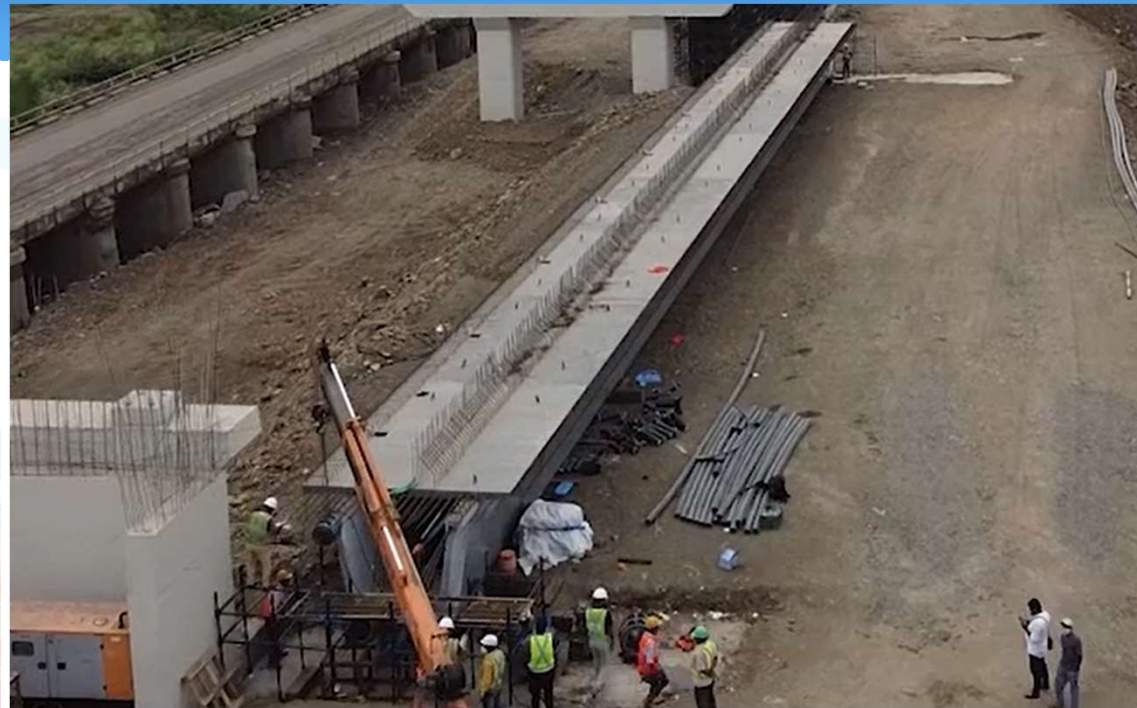
Alignment and Post-tensioning
