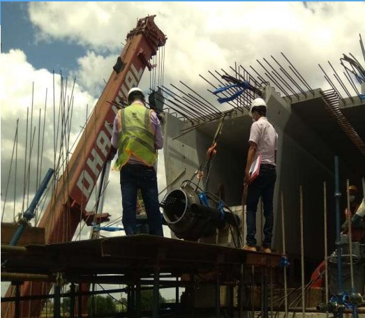
Alignment and Post-tensioning
