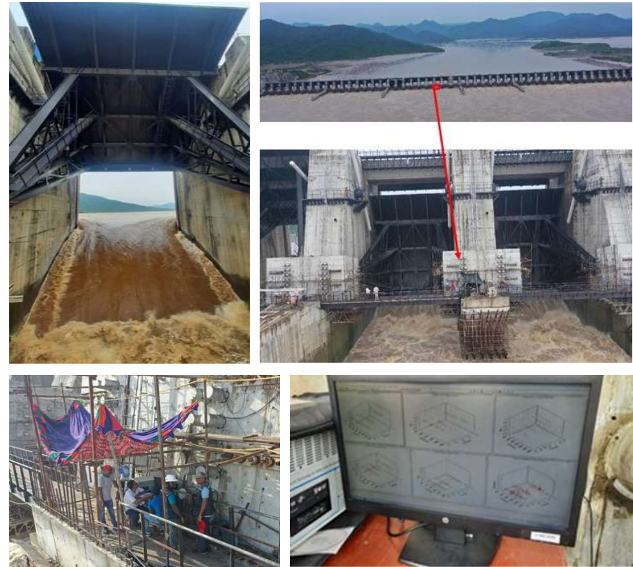
Prestressed trunnion beams in Polavaram Dam
