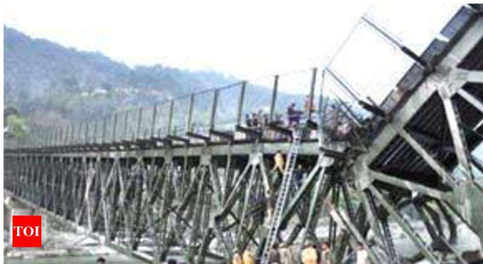
Bridge over Alaknanda river near Srinagar
