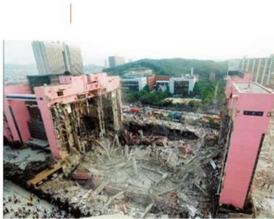
Sampoong Department Store Collapse due to Overload in Seoul, South Korea (1995).
