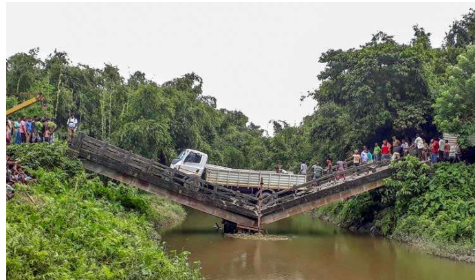
bridge collapse near Siliguri
