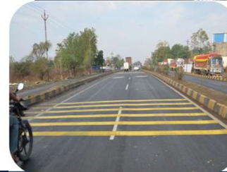
Transverse Bar Marking (TBM) Specification
