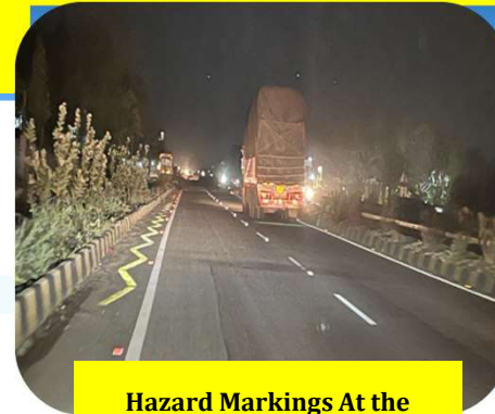
Hazard Markings At the Intersection Approach
