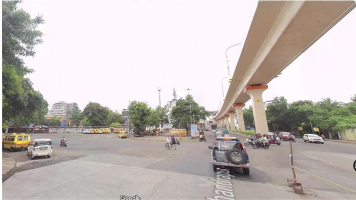
Improper traffic and pedestrian movements
