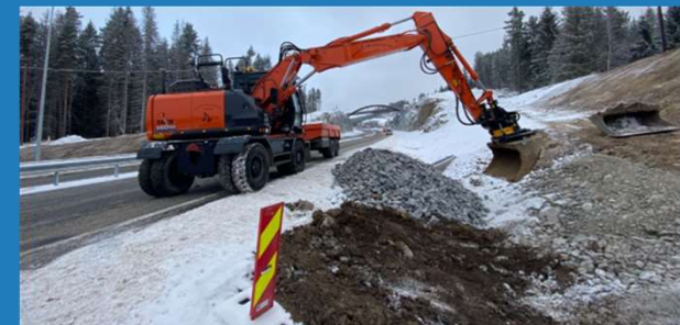
Photo: Per Kollstad / The Norwegian Public Roads Administration
