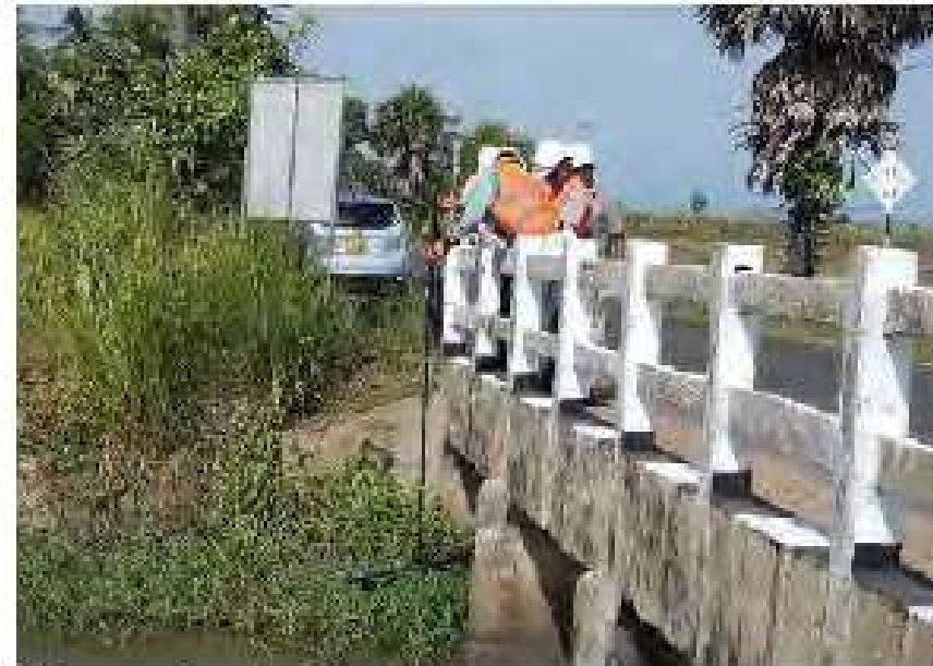
Inspection by Pole Camera
