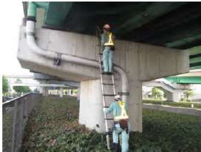
Inspection by Ladder
