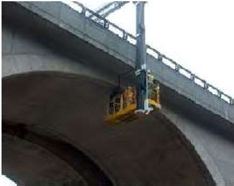
Inspection by Bridge Inspection Vehicle
