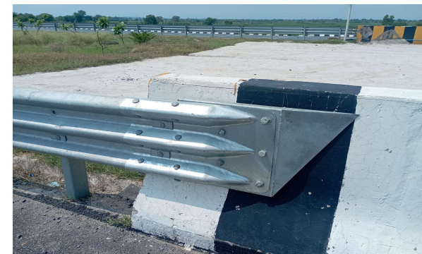
Barrier Installed Confirming to Performance Tests
