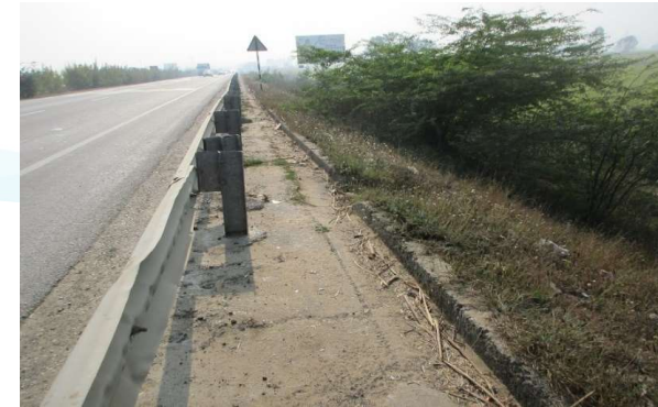
Barrier Installed Confirming to Performance Tests
