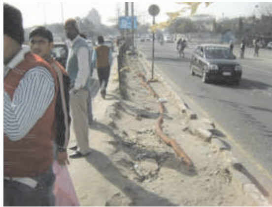
Audit of Existing Road (at site)
