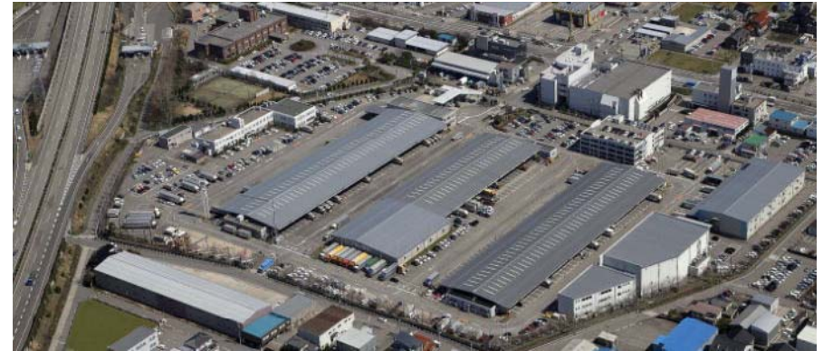
Truck terminal adjacent to interchange
