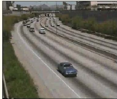
Reasonably free flow, Ability to maneuver is only slightly restricted, Effects of minor incidents still easily absorbed
