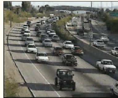
Operation near or at capacity, No usable gaps in the traffic stream, Operations extremely volatile, Any disruption causes queuing
