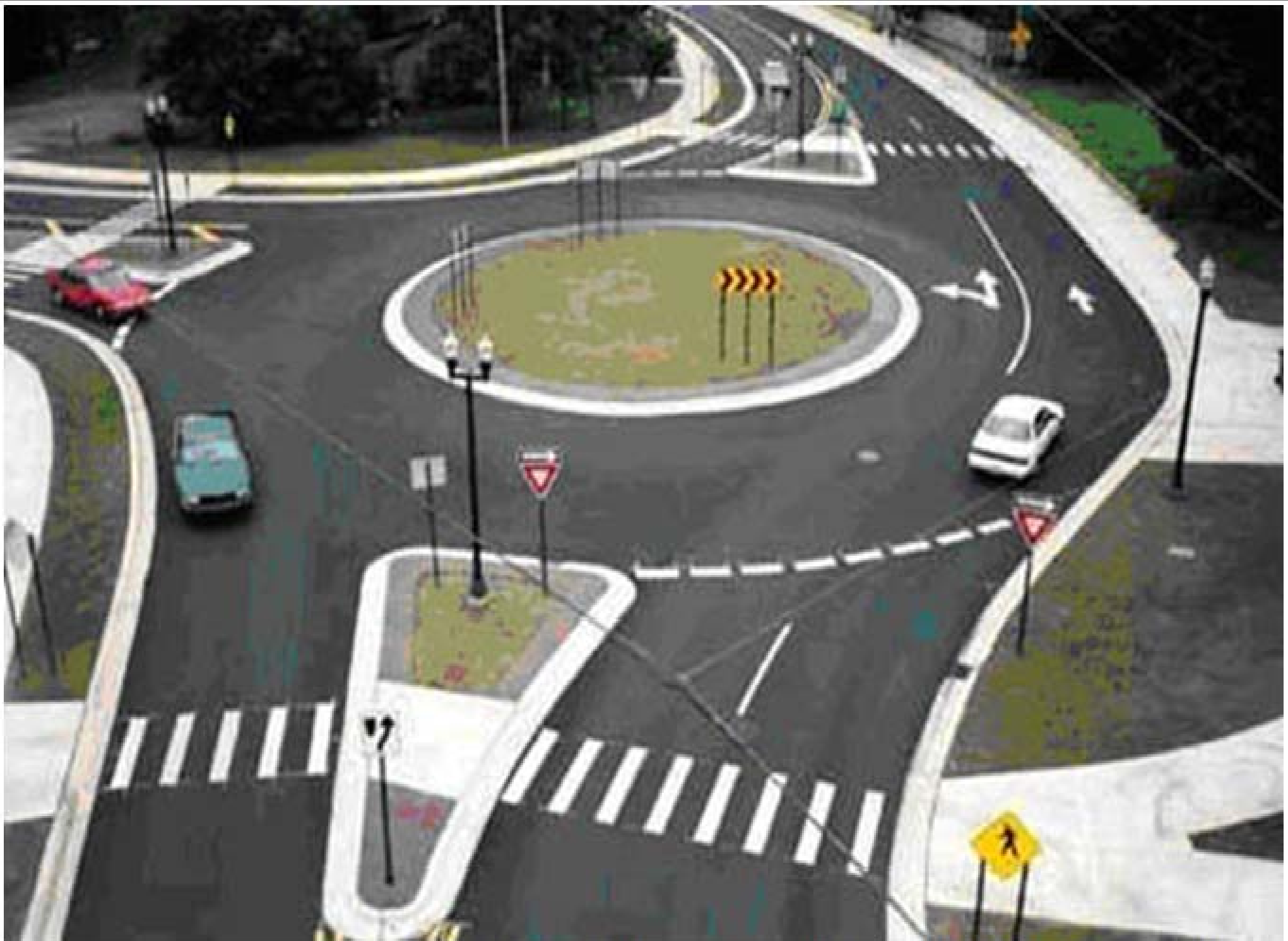
Image Courtesy of Ingham County Road Commission
