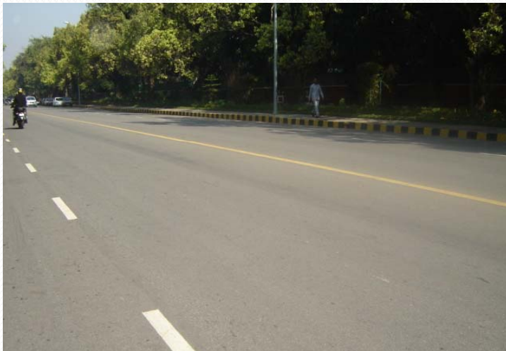
Rajaji Marg ( SDBC + Microsurfacing) , Jan'08
