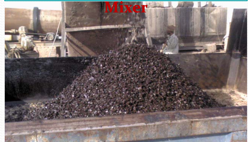
Discharge of Cold Mix to Dumper
