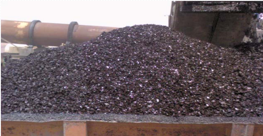
Production of cold mix for SDBC
