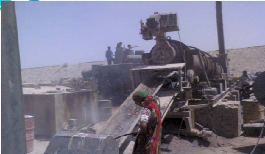
Adding Pre-mix Water
