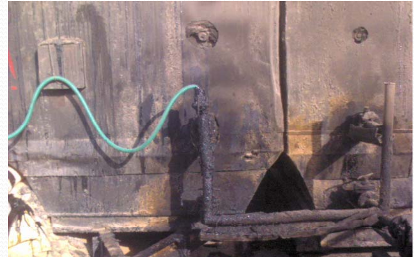
Adding Emulsion in Drum Mixer
