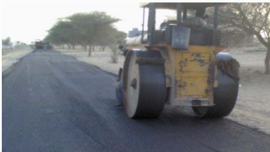
Compacting cold mixed SDBC
