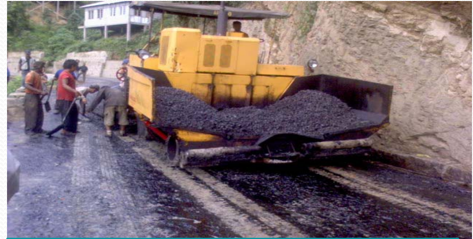
Laying of cold BM with emulsion at Aizawl
