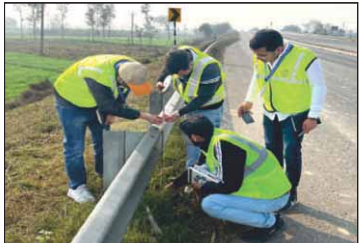
Project Team measuring height of Metal Beam Crash Barriers
