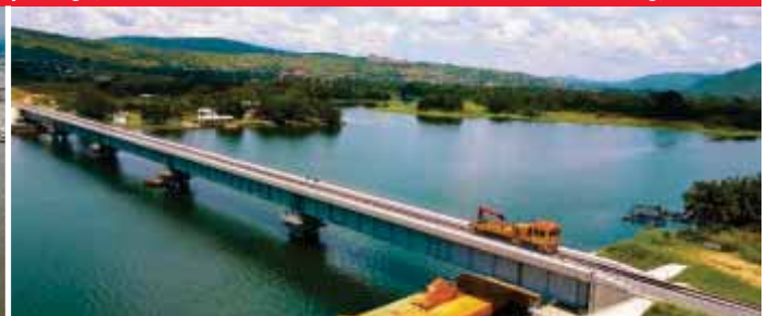
Volta Bridge, Tema-Mpakadan Railway, Ghana
