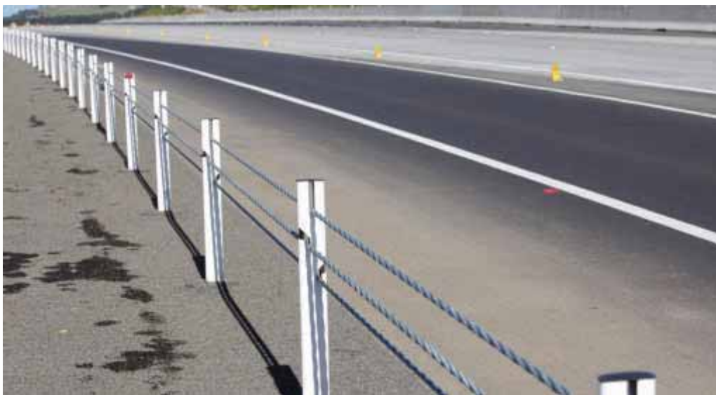
FIG 2 Forgiving roads with crash barrier
